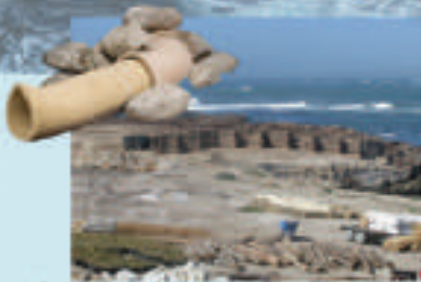
Construction of pipes and early nest restoration. (Photo credit: Oikonos)
